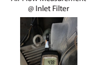
Inlet Air Conditions Measurement
