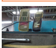
Air Flow Measurement @ Inlet Filter
